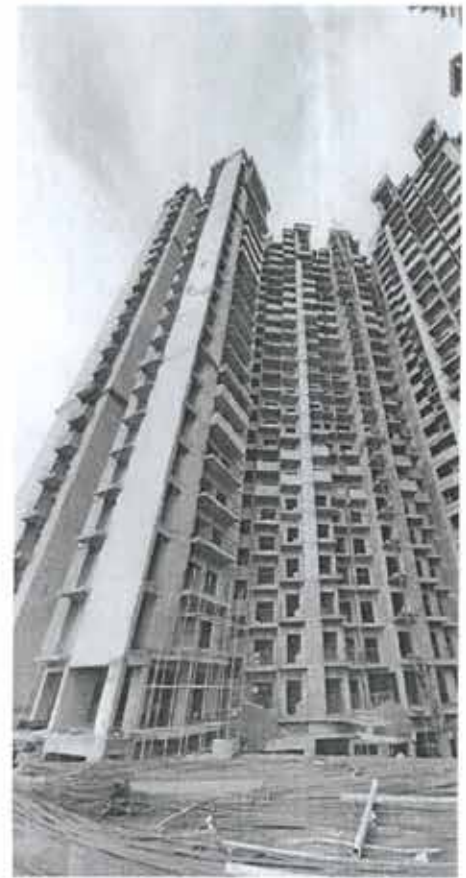
TOWER B-5 SIDE
