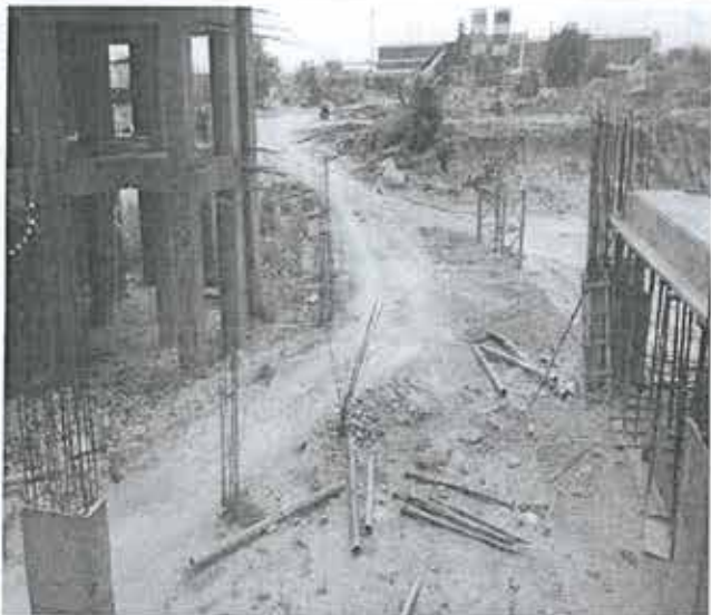
T-11 NONTOWER AREA
