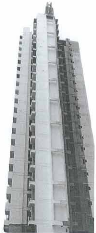
TOWER T-7 SIDE
