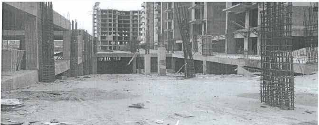
RAMP WITH NON TOWER BETWEEN TOWER-T6 & TOWER-T7
