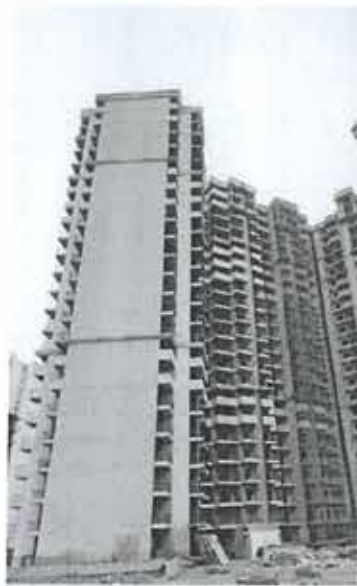
TOWER B-1 REAR
