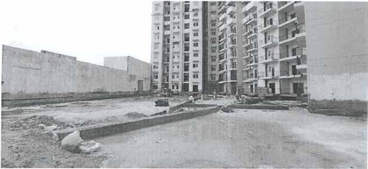
LANDSCAPE WORK OVER STP
