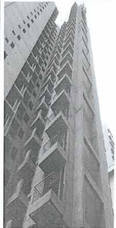
TOWER T-9 SIDE
