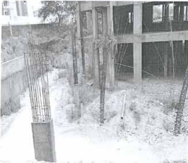
T-10 NONTOWER AREA
