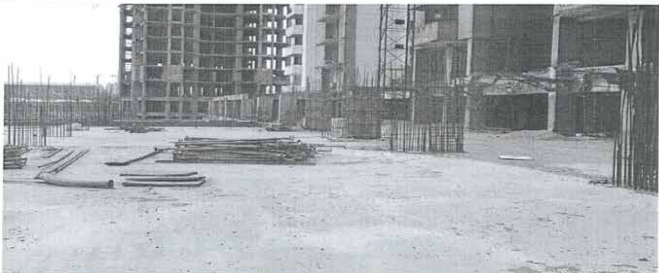
TOWER T-4 TO T-6 REAR SIDE NON TOWER CENTRAL AREA
