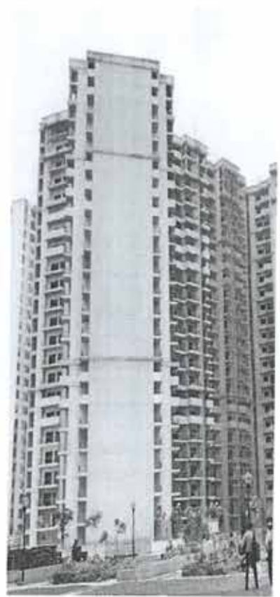
TOWER B-1 SIDE
