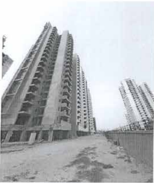
TOWER T-6 TO T-4 NONTOWER AREA
