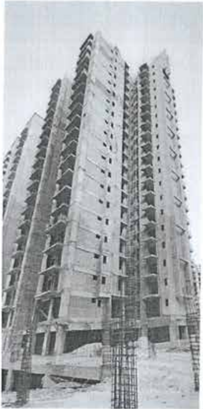
TOWER T-6 SIDE
