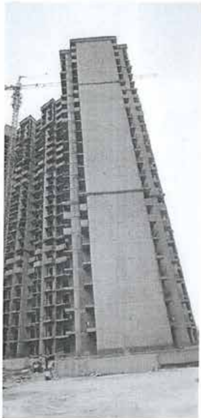
TOWER B-4 REAR
