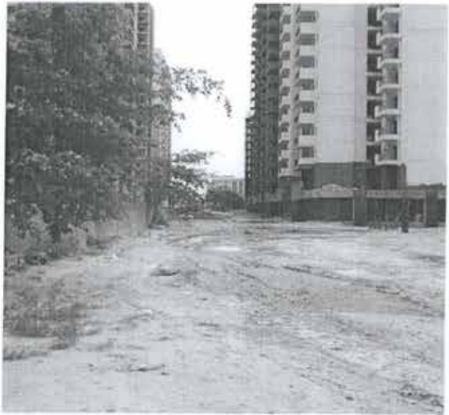
TOWER T-7 TO T-9 NONTOWER AREA
