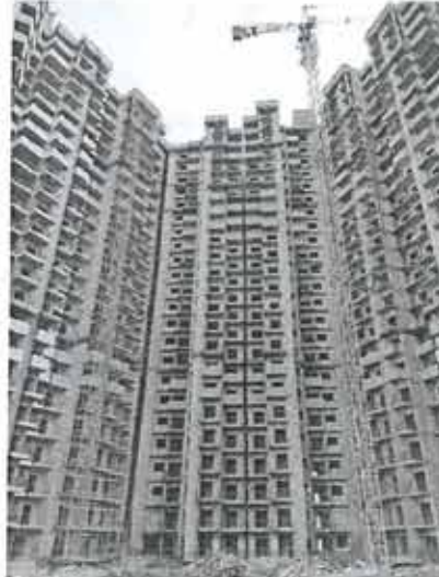
TOWER B-2 REAR
