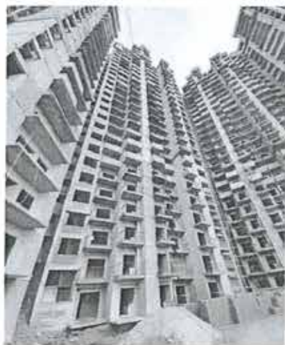
TOWER B-3 REAR
