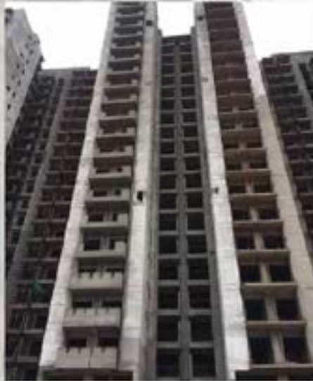
TOWER T-8 REAR
