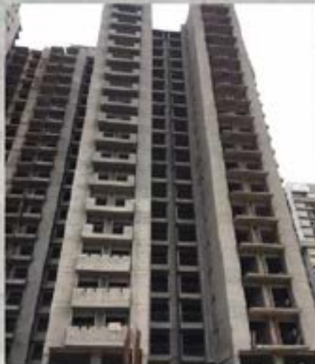
TOWER T-9 REAR
