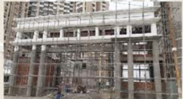
FRONT GATE NO. 1
