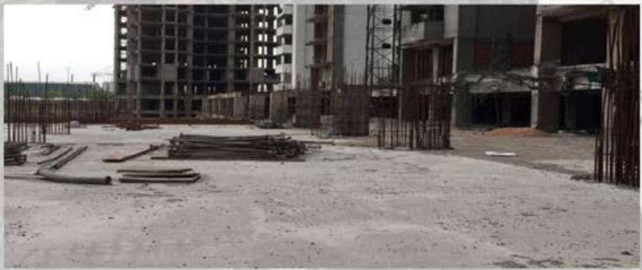
TOWER T-4 TO T-6 REAR SIDE NON TOWER CENTRAL AREA
