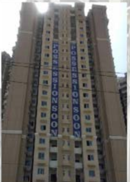
TOWER A-4 FRONT
