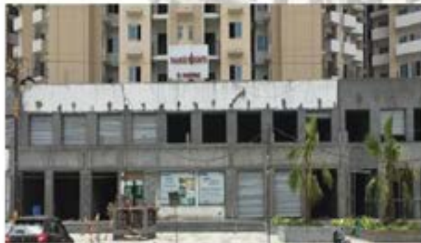
COMMERCIAL SHOPS FRONT
