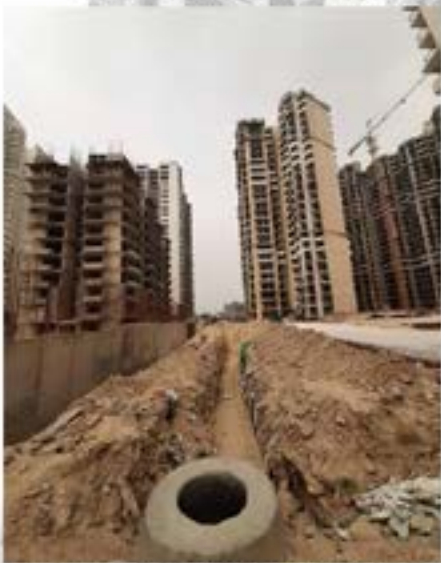
SEWER WORKS NEAR A-1
