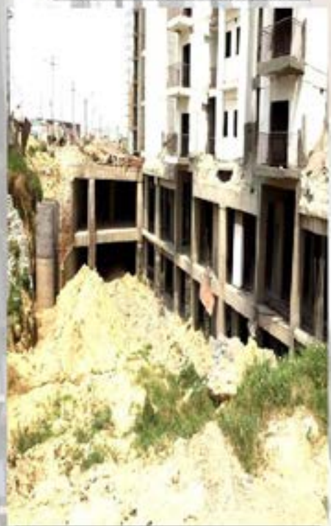
TOWER B-6 NON TOWER AREA
