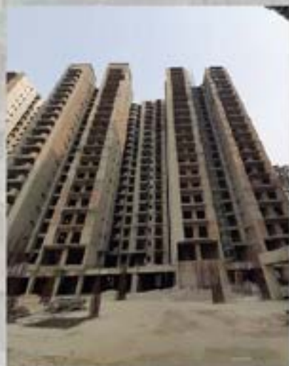
TOWER T-6 REAR
