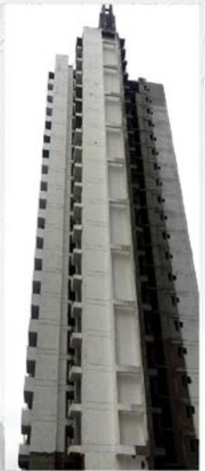
TOWER T-7 SIDE
