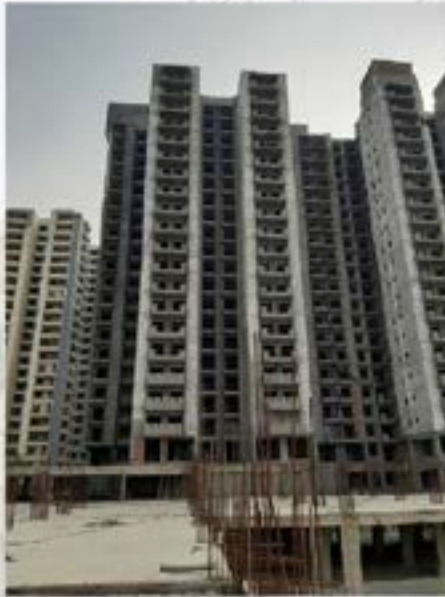
TOWER T-7 REAR
