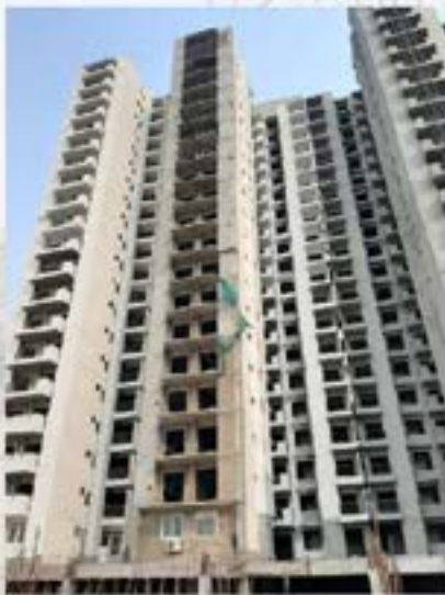
TOWER T-4 REAR
