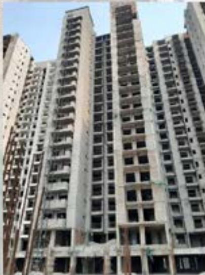
TOWER T-5 REAR
