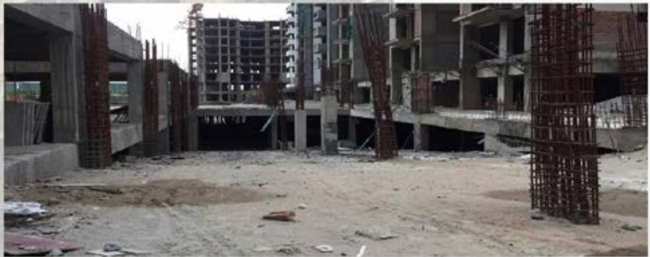
RAMP WITH NON TOWER BETWEEN TOWER-T6 & TOWER-T7
