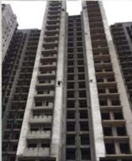
TOWER T-8 REAR
