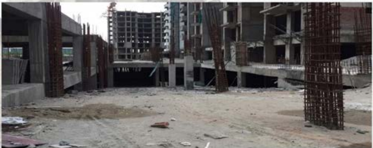
RAMP WITH NON TOWER BETWEEN TOWER-T6 & TOWER-T7
