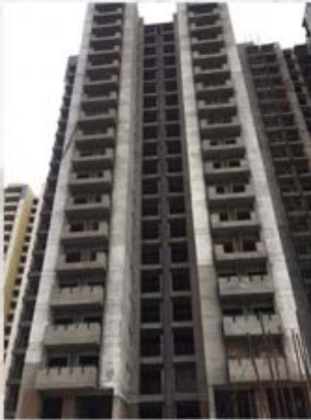
TOWER T-7 REAR
