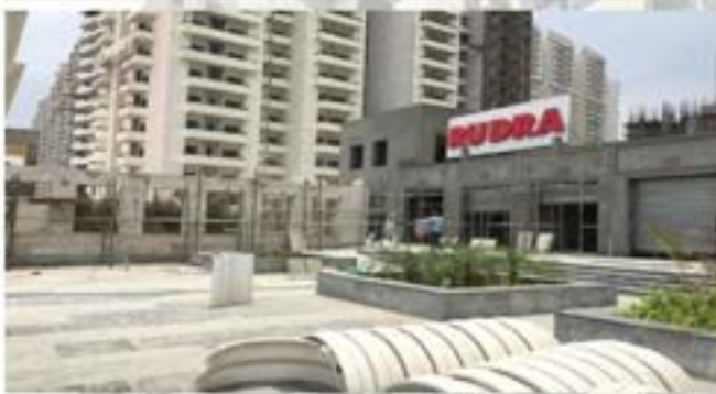
FLOORING WORK IN PROGRESS
