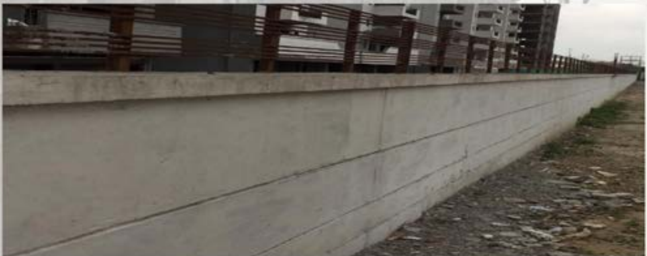
BOUNDRY WALL WORK ON PROGRESS
