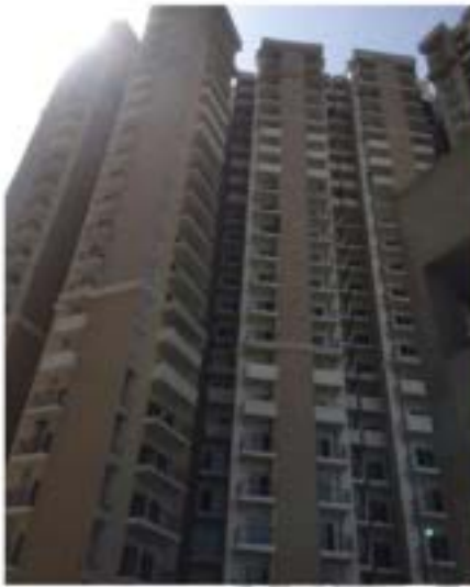
TOWER A-1 FRONT
