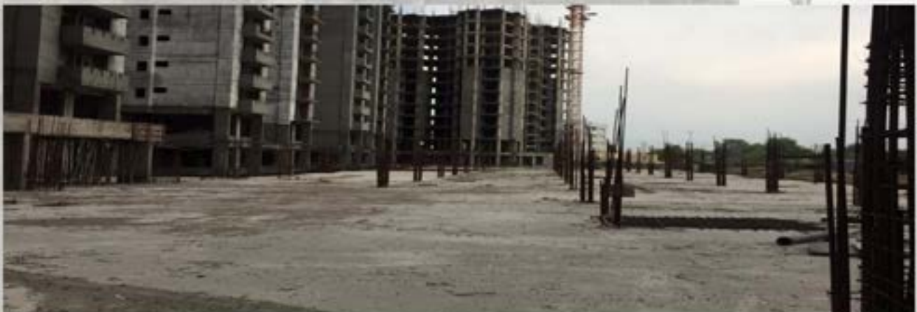
T-7 TO T-9 REAR SIDE NON TOWER CENTRAL AREA COLUMN CASTING ON PROGRESS
