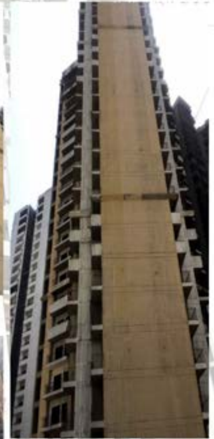
TOWER B-1 SIDE
