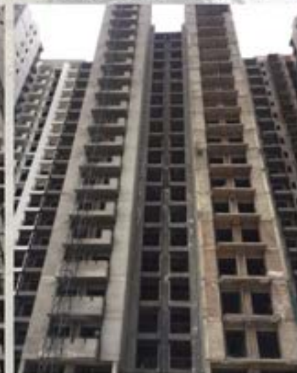
TOWER T-5 REAR
