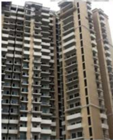
TOWER A-3 FRONT
