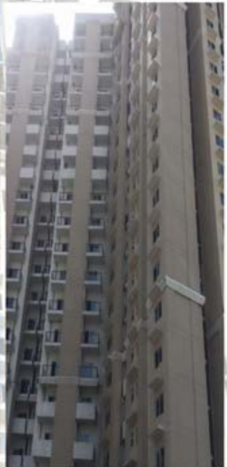
TOWER A-2 FRONT
