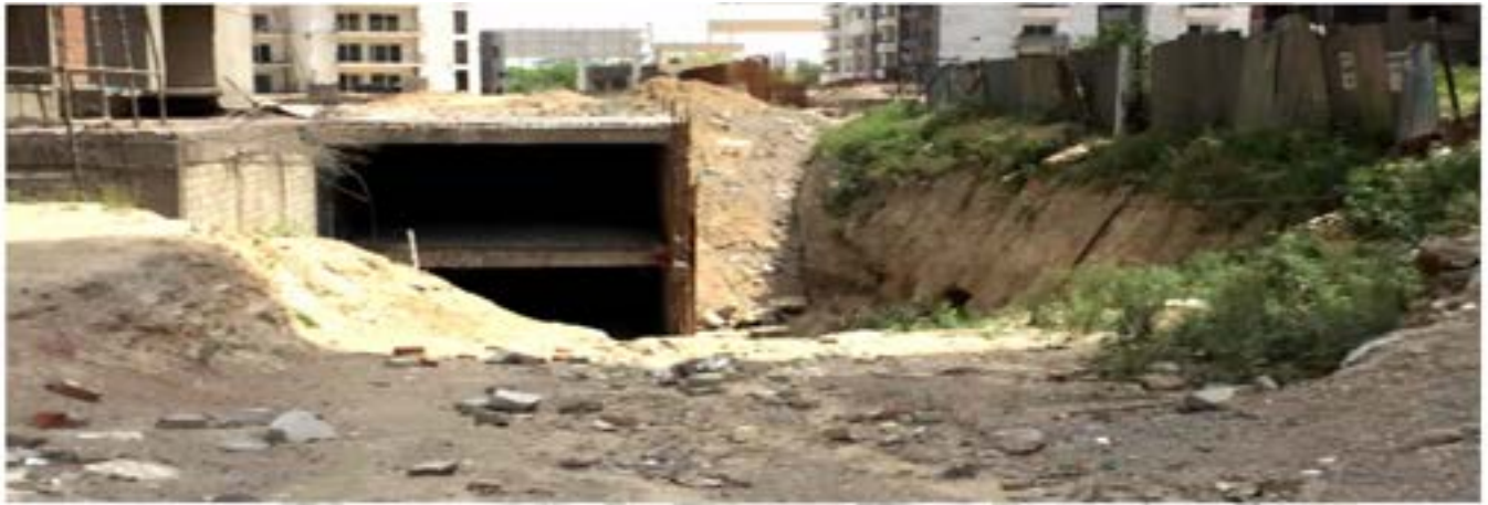
PART 9 TOWER B1 SIDE NON TOWER AREA
