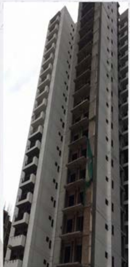
TOWER T-4 REAR
