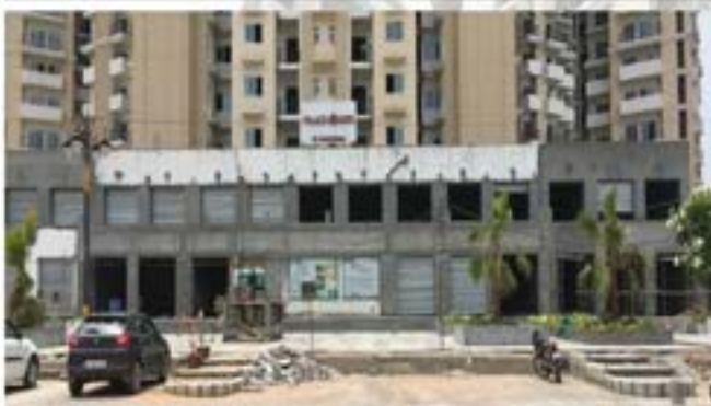
COMMERCIAL SHOPS FRONT
