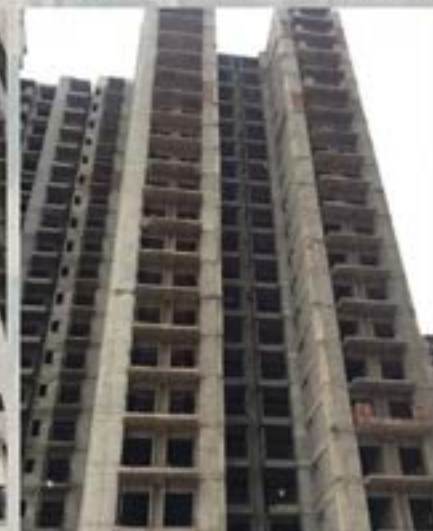
TOWER T-6 REAR
