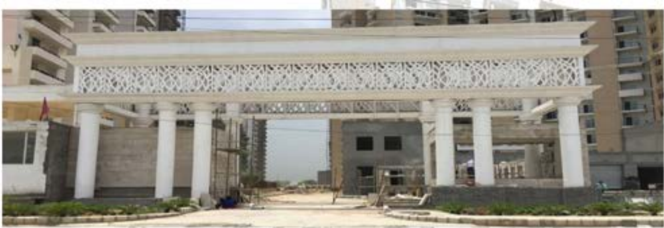
FRONT MAIN ENTRANCE GATE CONSTRUCTION ON PROGRESS
