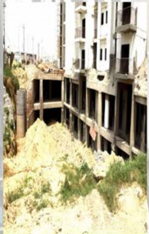
TOWER B-6 NON TOWER AREA
