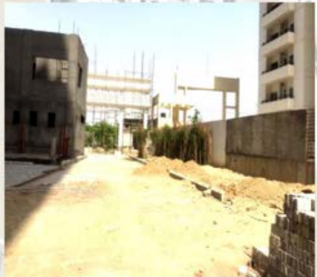
REAR SIDE GATE AREA
