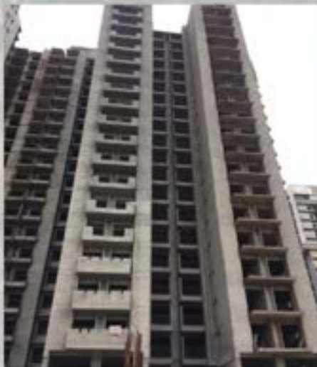
TOWER T-9 REAR
