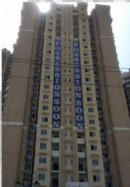
TOWER A-4 FRONT
