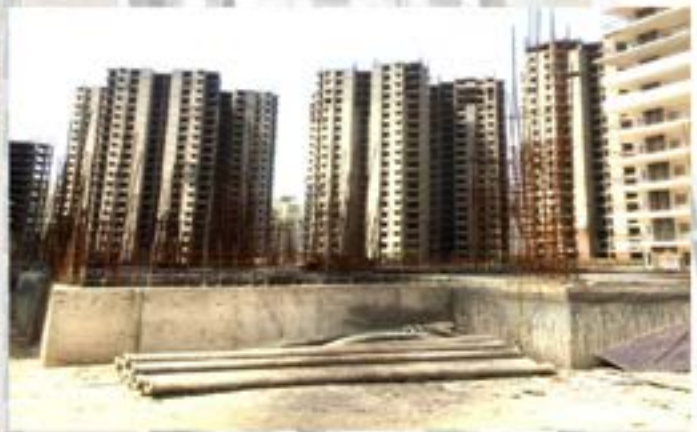
CLUB AREA SLAB CASTING
